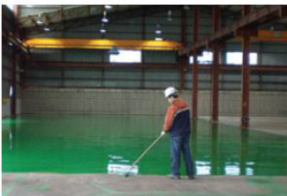
APPLYING TOP-COAT
